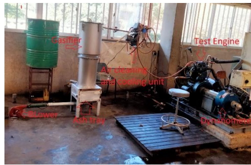
Figure 5. Gasification system and Test engine layout
