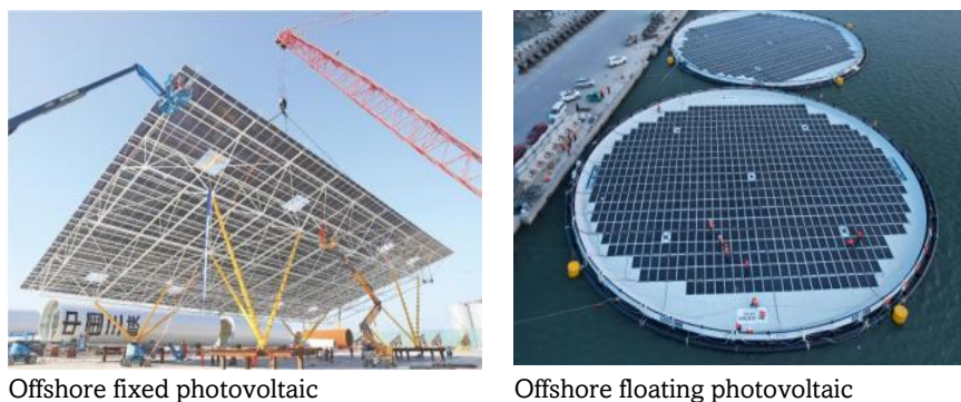
Figure 5 Structural forms of offshore photovoltaic
